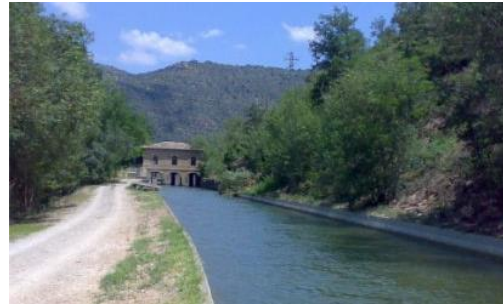
Flowing waters | River dams | Irrigation
