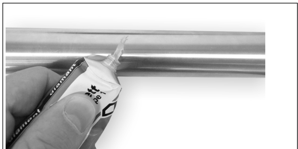
Fig. 1 using coupling grease
