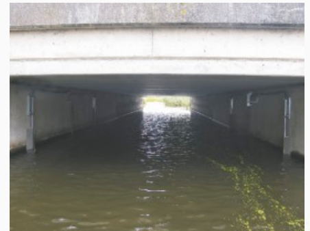
View of measurement place
