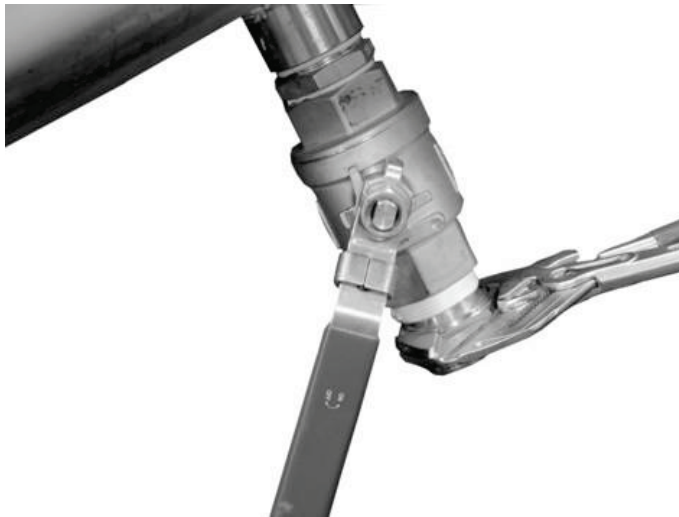
Fig. 13-31 Fixing the sensor screw connection to the stop ball valve
