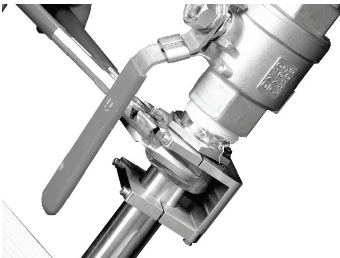
Fig. 13-37 Unscrew the spigot nut for sensor removal
